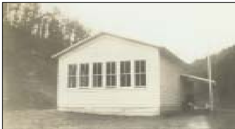
The newly remodeled Three Mile School in the fall of 1935.
